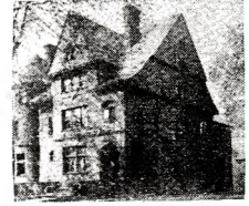
Front View Conservatory Bldg.
